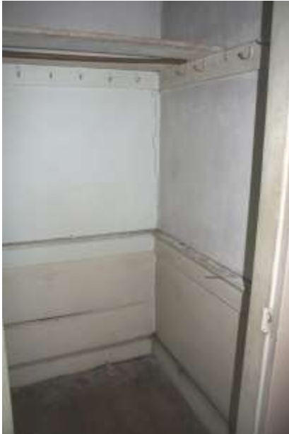
Room 201, Closet Interior
