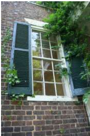
First floor 9/9 windows Second floor 6/9 sash windows
