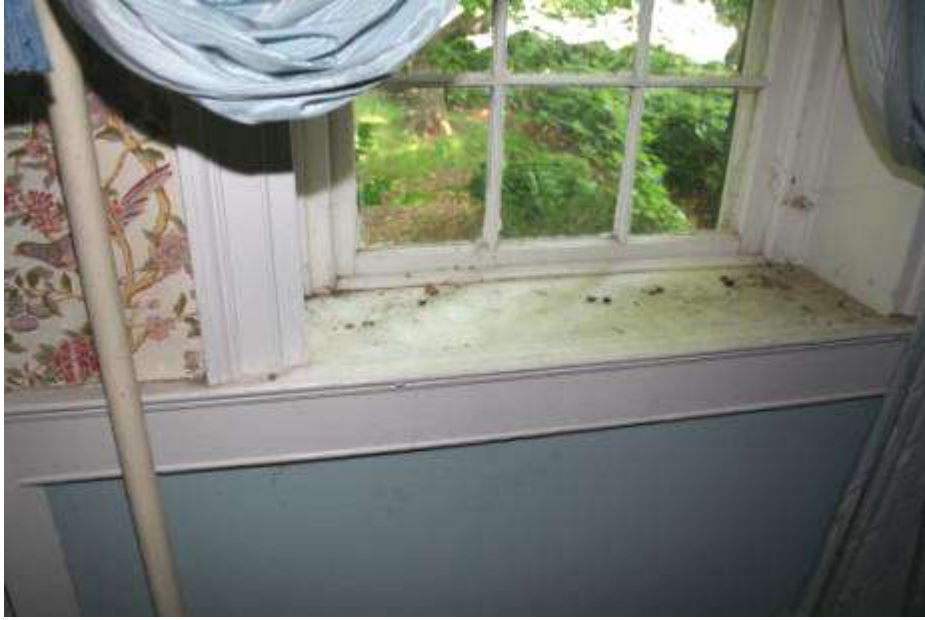
Room 102, west wall, window 1, including the surbase
