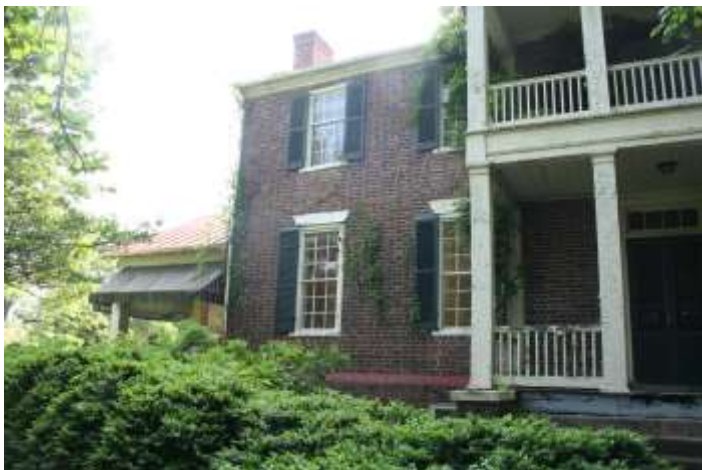
West Elevation, north end
