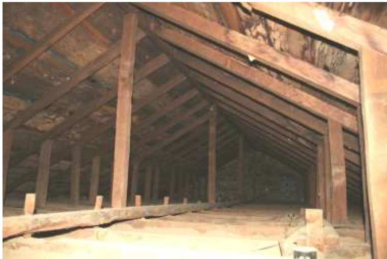
View to north
