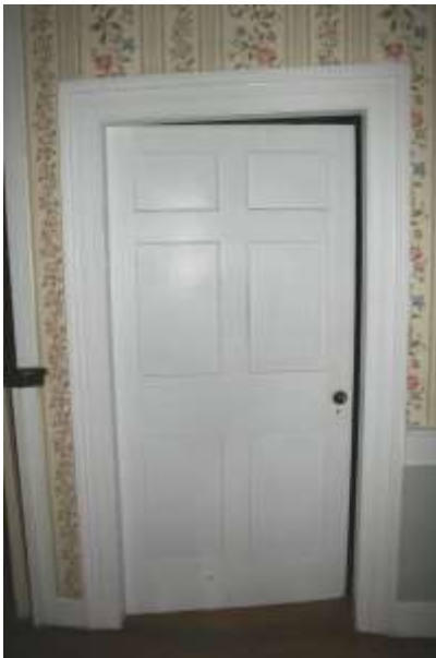
Door on west wall of Room 200
