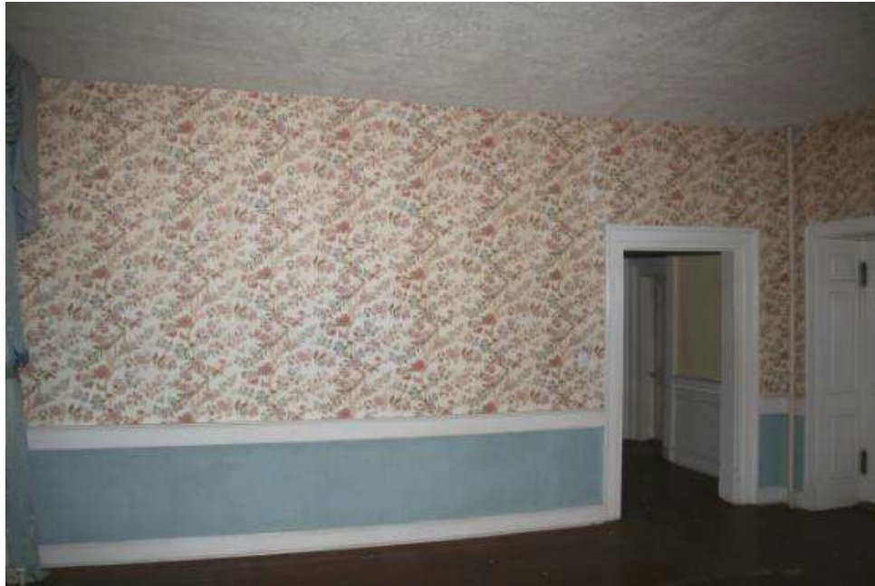
Room 102, north wall, door 1
