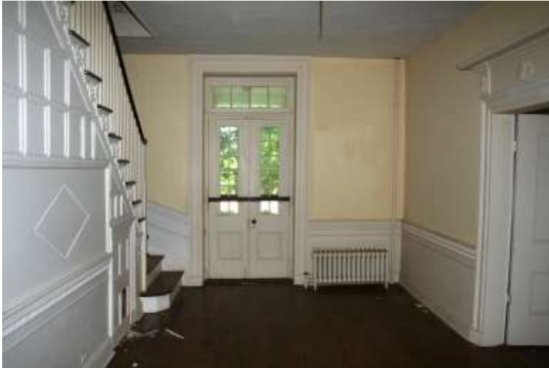
Room 100, View west
