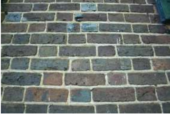
Typical water-struck brick
