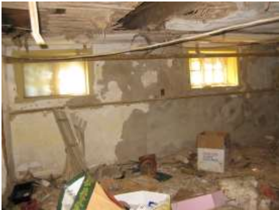
Room 002, windows on west elevation
