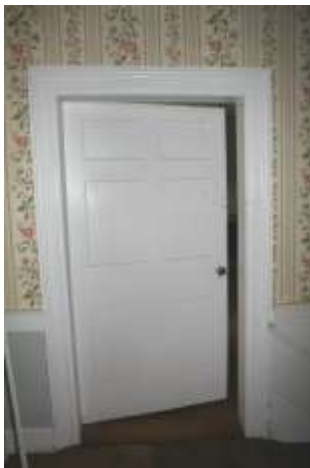
Door on south wall
