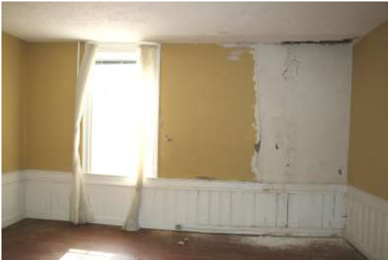
Room 101, east wall
