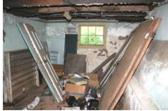
View west with chimney on right
