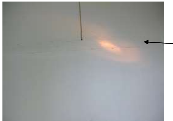
Room 205, Ghost mark of wall trim
