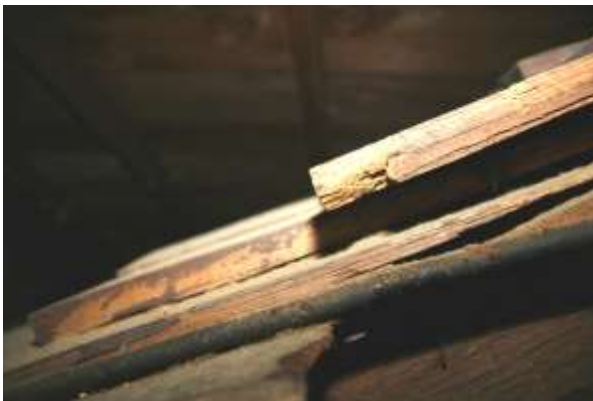
Second period shingles encapsulated in west portico pediment roof. Note red paint on shingle in left photo.
