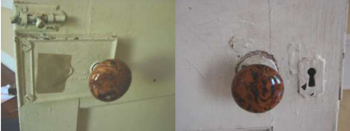
Room 202 left: rimlock and bolt on inside; right: current handle and ghost of previous lock
