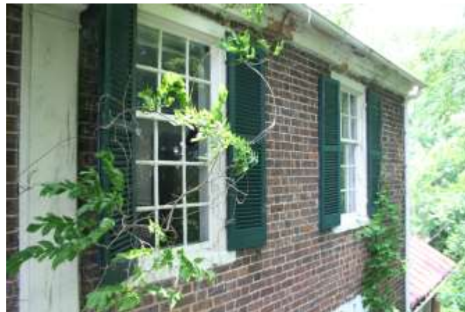
First floor 9/9 windows Second floor 6/9 sash windows
