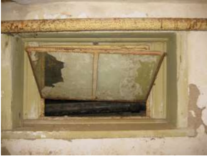
Room 002, window on east wall
