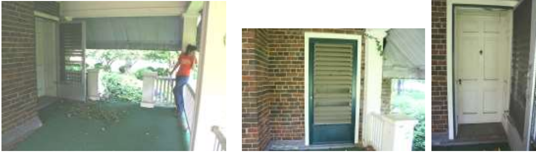
North porch with door added for access
