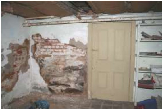
Room 003 East Wall
