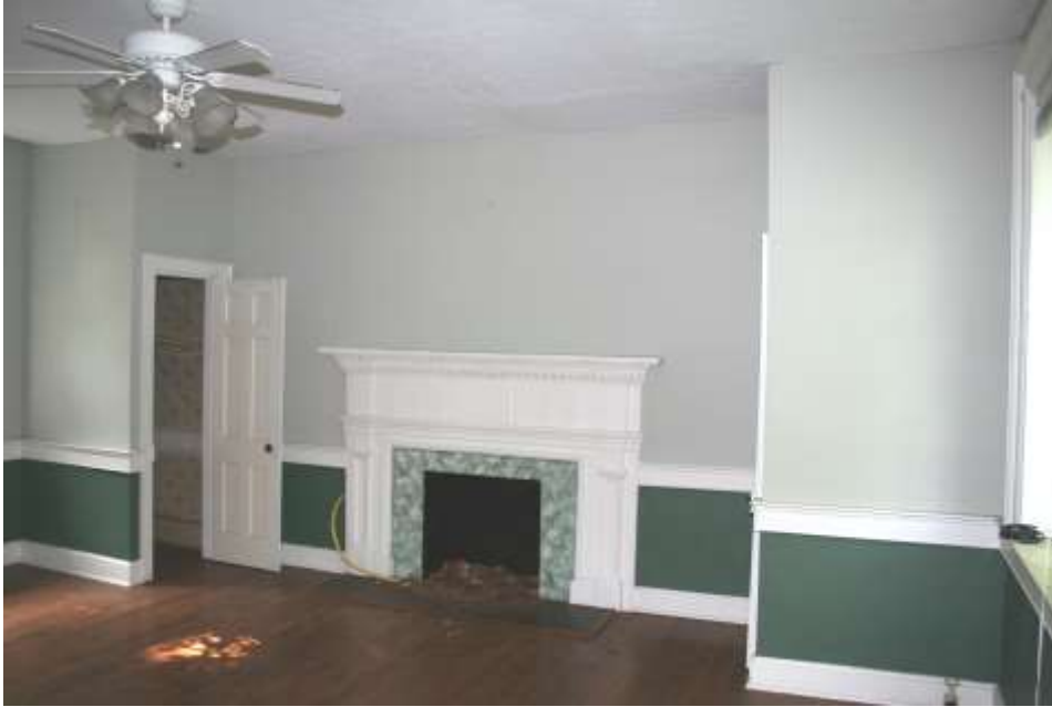
204, south wall with added closets
