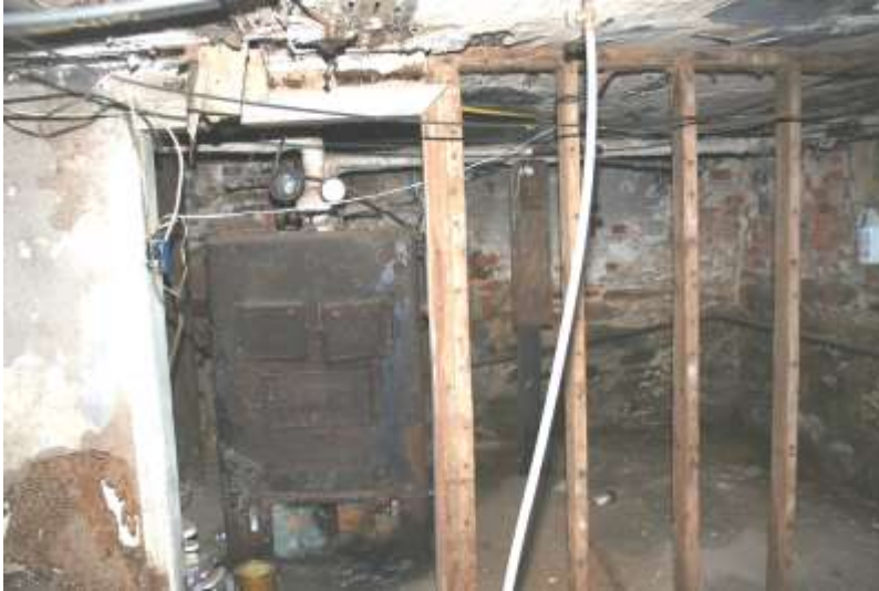
Room 004, furnace and partition
