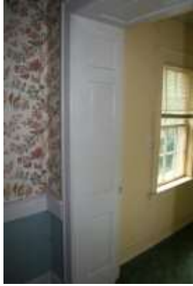
Room 102, door 3 revealing paneling in door jamb
