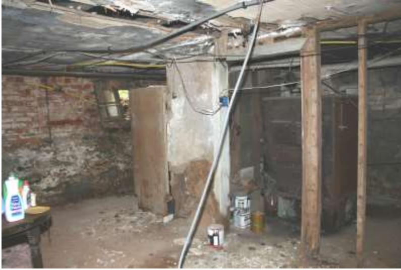
Room 004, southeast corner
