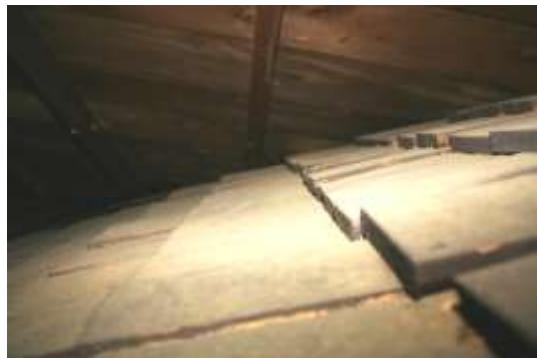
Second period shingles encapsulated in west portico pediment roof. Note red paint on shingle in left photo.
