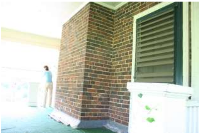
Original north wall and chimney
