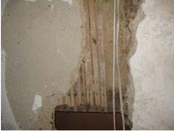
Room 002, ceiling – a more modern plaster on wire lath
