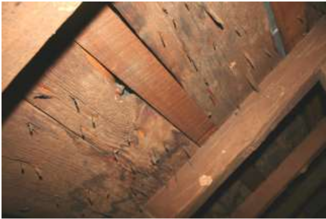
Sheathing on rafters; supplemental modern board
