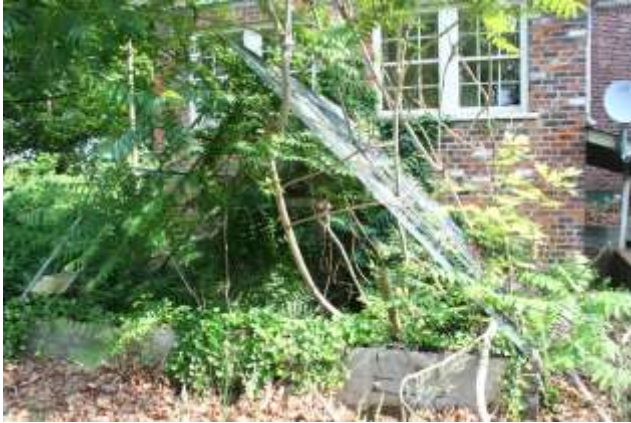
Greenhouse, south elevation
