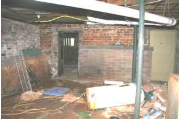
Room 006 View west
