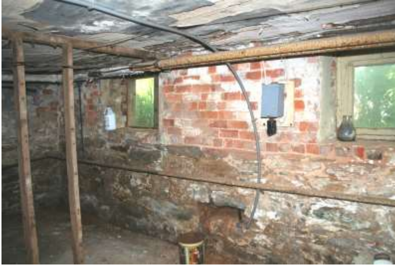
Room 004, windows on west wall
