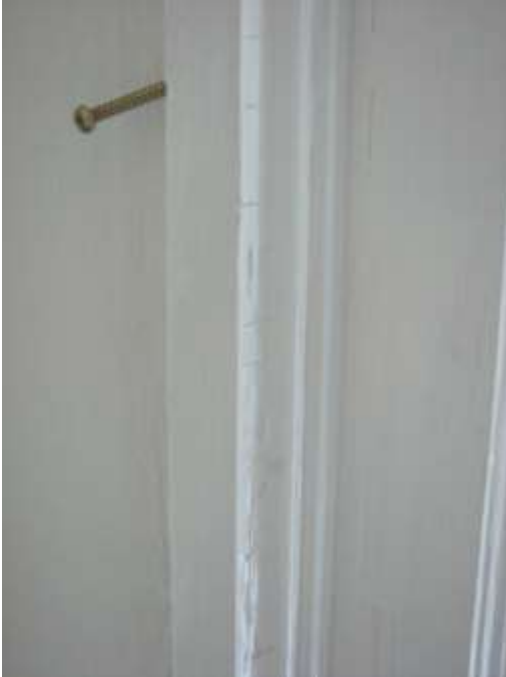
Room 203 window architrave, east wall
