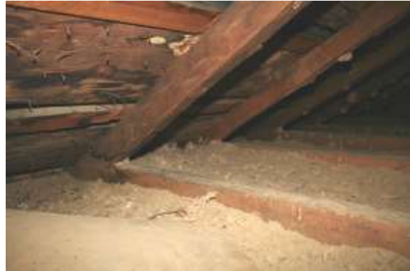
Rafters align with joists
