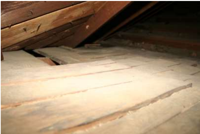
Shingles of west roof slope preserved under west portico pediment roof
