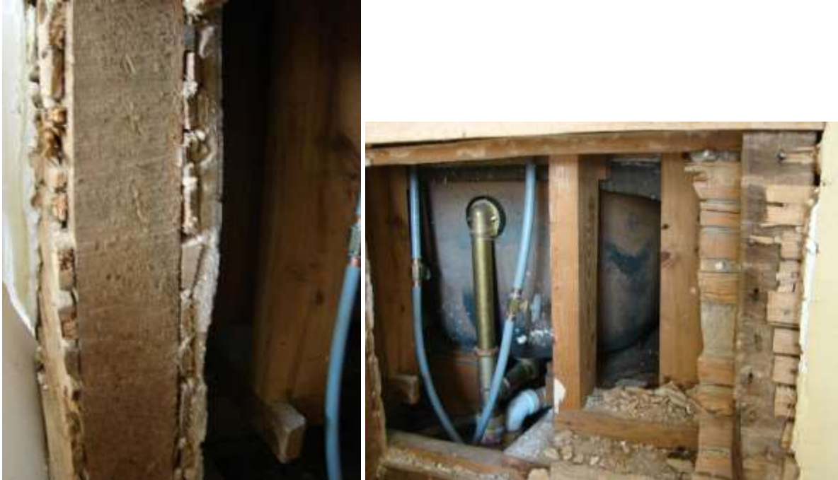
Room 202 East wall, open panel with lath and plaster
