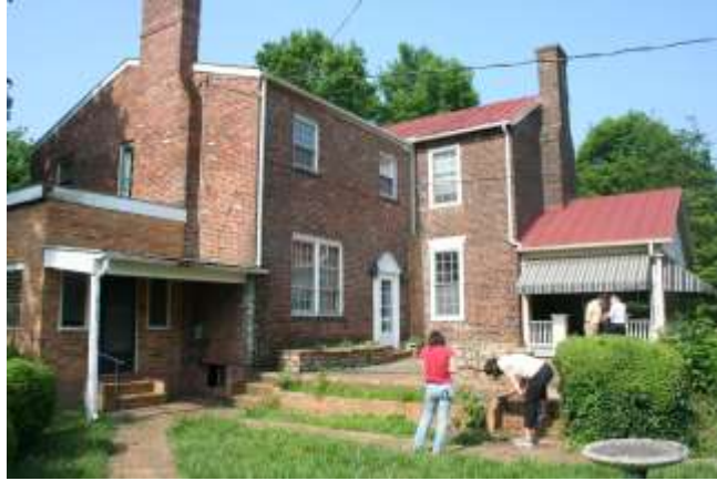
Rear of First Addition
