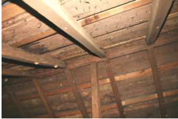
Rafters mortise into ridge board
