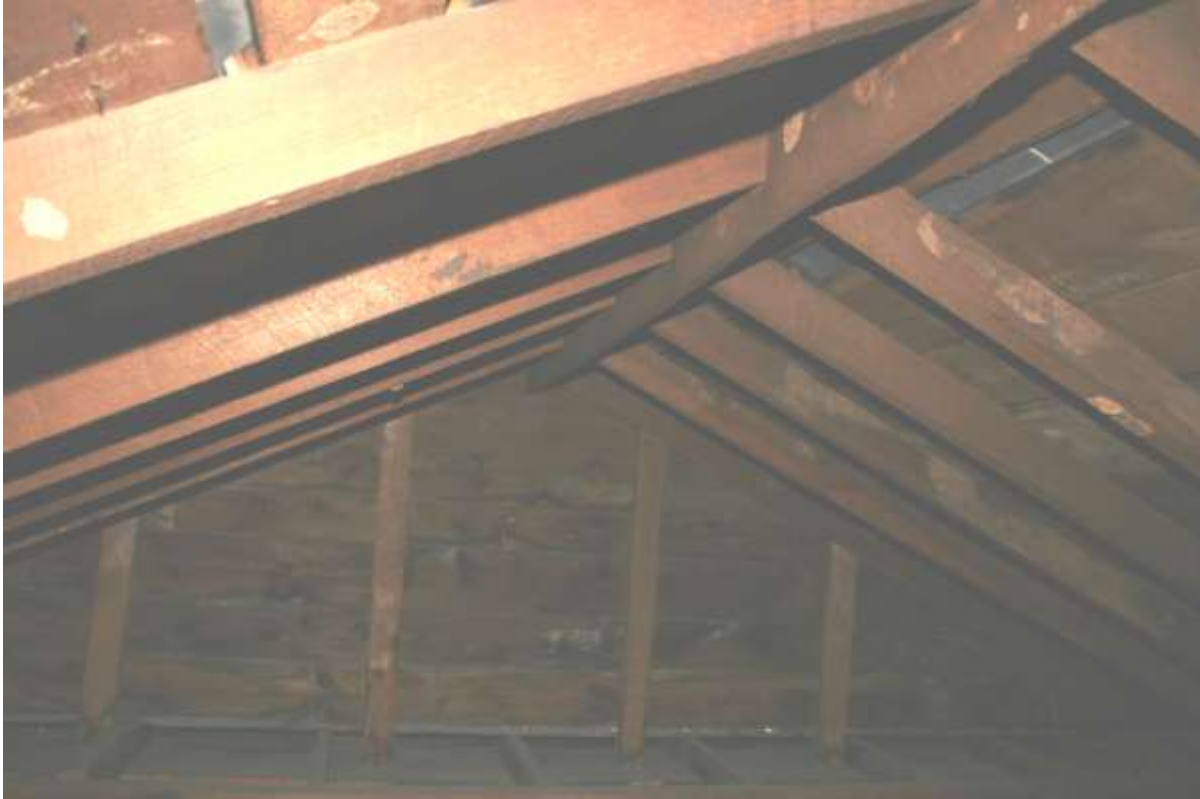
Attic framing of west portico
