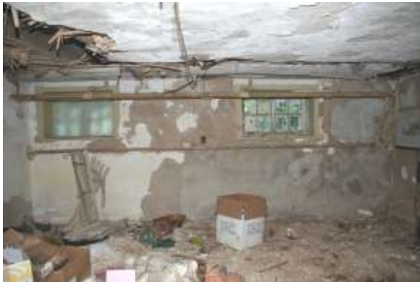
Room 002 View west
