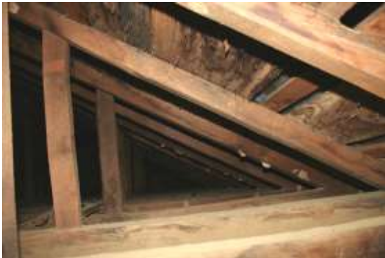
Posts supporting rafters
