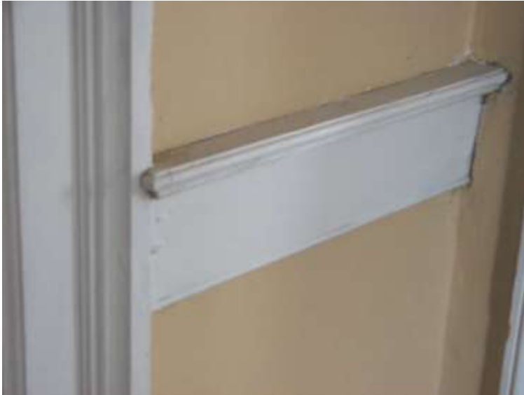
Room 204, surbase on south wall fitted into south door trim
