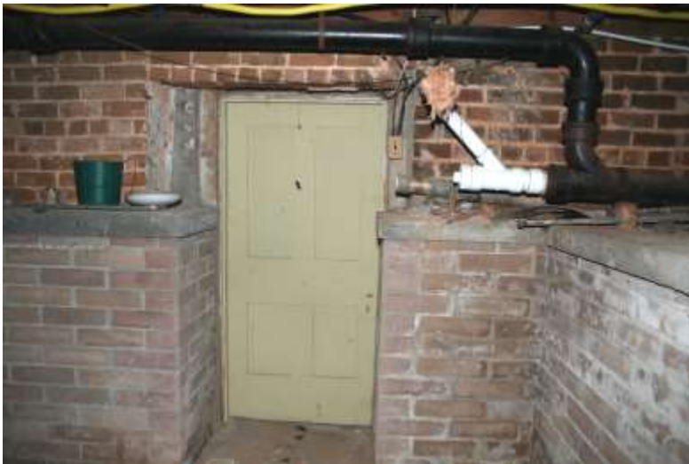
Room 006 Door connecting to Room 003.
