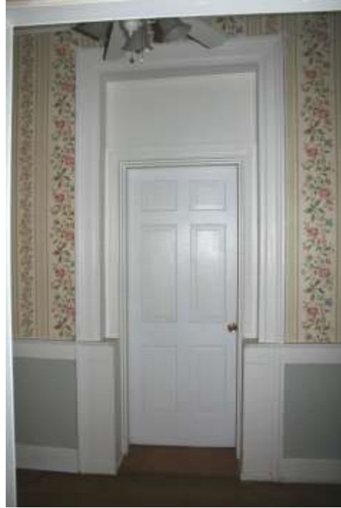
east wall, originally a window
