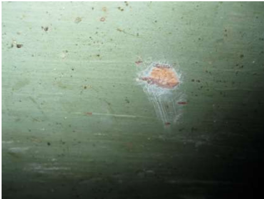
(Figure 3, attic wall)
