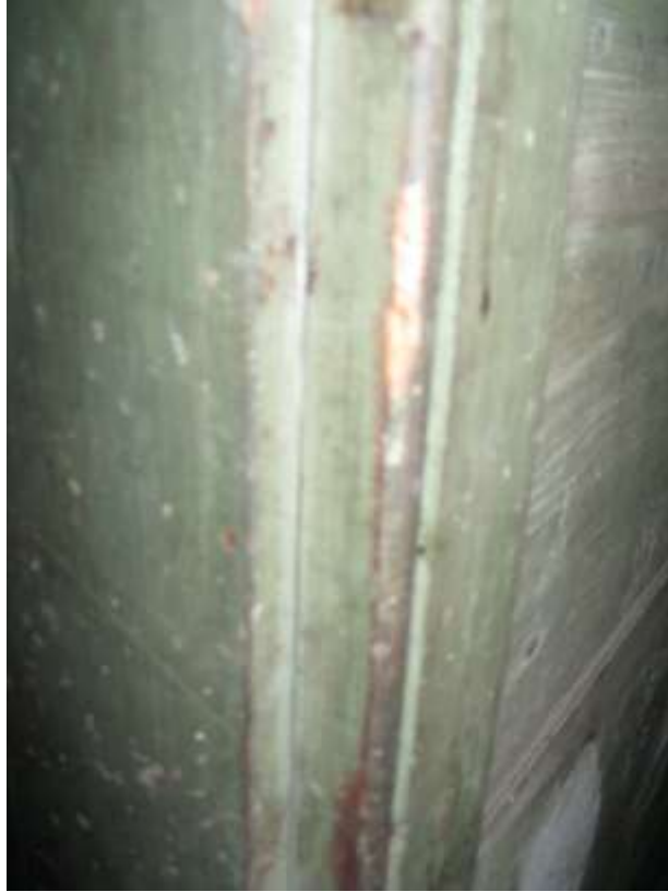
(figure 4, attic wall)
