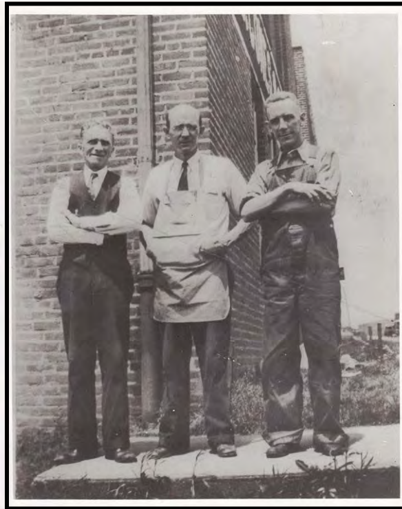
Figure 4. John Niehaus (center) in front of the Dewitt-Wharton Building, undated photo
