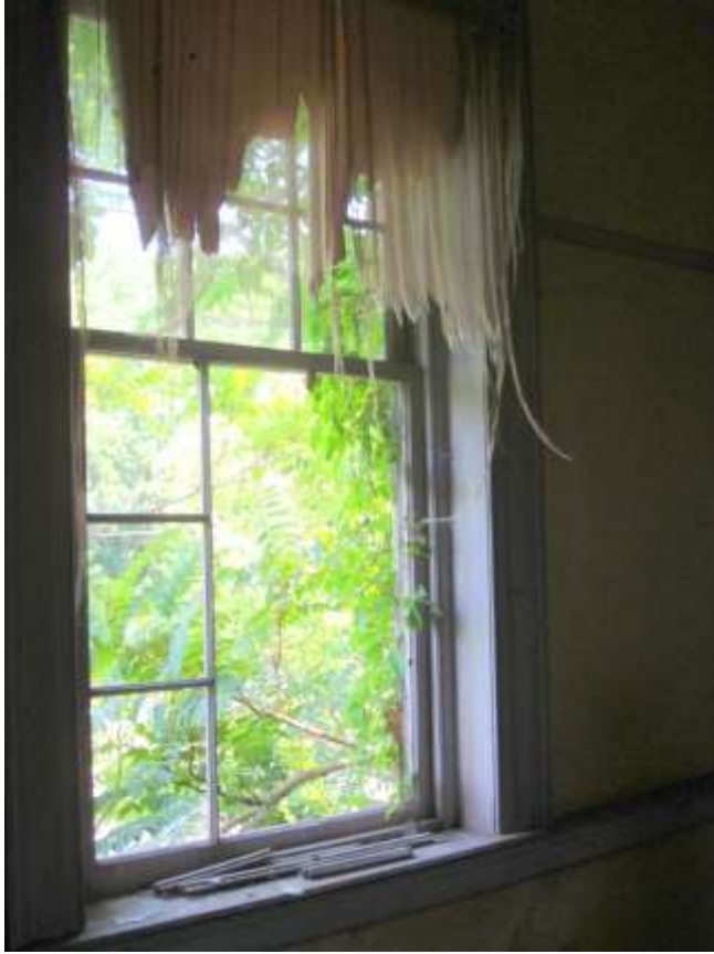
(Rm. 201) North Wall Window
