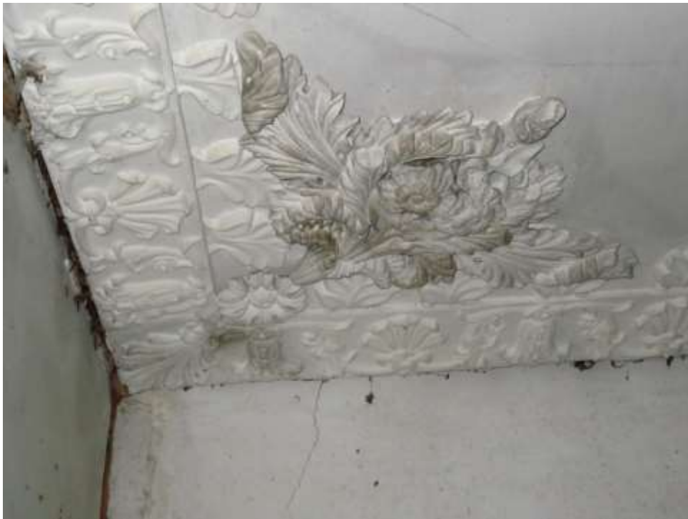
(Rm. 101) Plaster Moulding Detail on Corners of Ceiling
