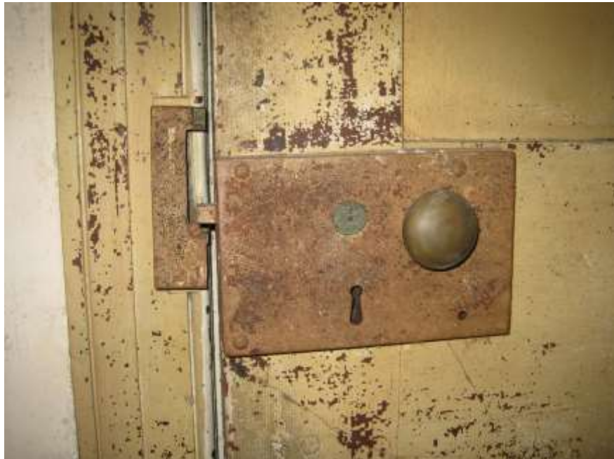
Figure X. (KF picture) Oakland, Room 202, door D-E-01 showing trim, lock and keeper and painted finish. Note that lock is installed correctly
