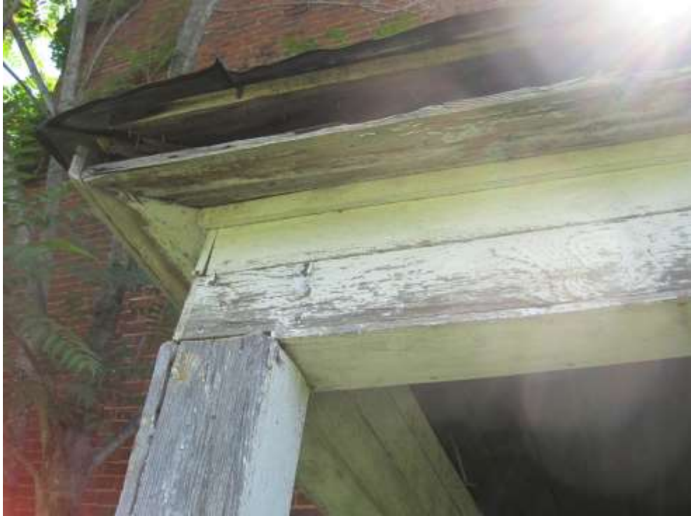
Figure X. (KF picture) Oakland, west elevation, showing porch column, trim, and roof construction details.
