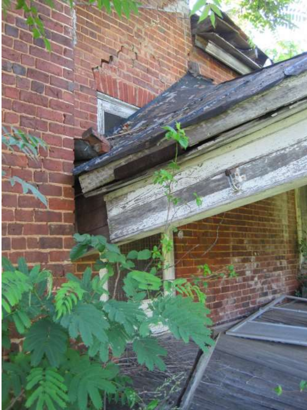
Figure X (KF Picture): Oakland, west elevation showing Door-W-01 access to porch, elevation of sill plate; brick arch construction over doorway; paint ghost showing original placement of porch roof; and cornice construction of porch.
