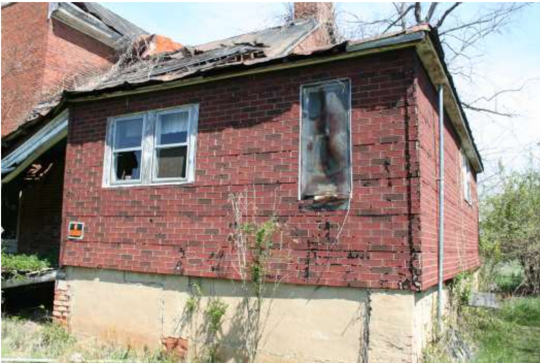
Figure X (TM Picture ): Oakland, west and east elevation of Section 3 showing change in materials, roofline, and construction..
