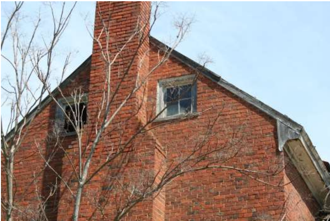
Figure 2: (TM Picture ) Oakland, west elevation, showing chimney, attic windows, eave trim and cornice.
