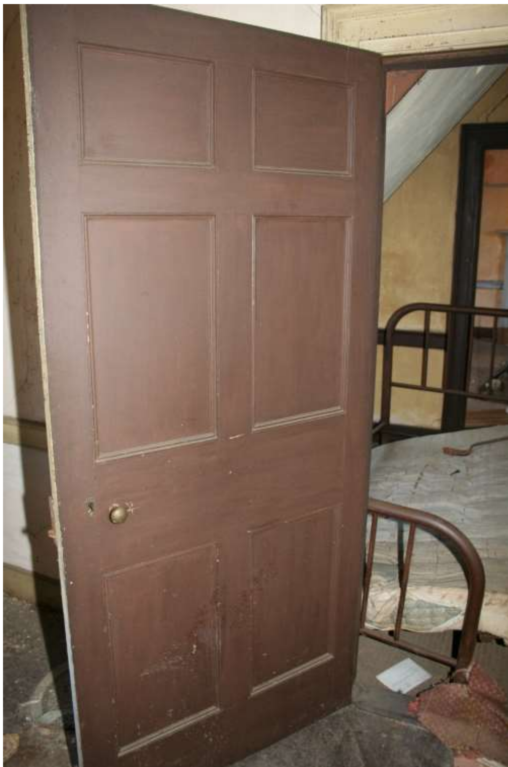
Figure X. (TM picture) Oakland, Room 202, hall face of door D-E-01 showing flat recessed panels, hardware, color and trim.
