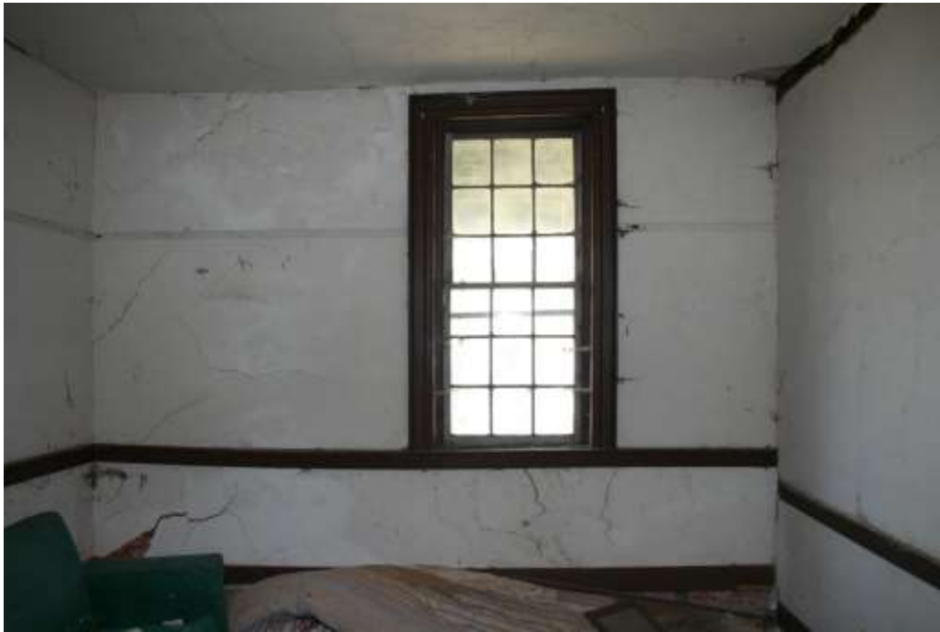
Figure X: (TM Picture) Oakland, Room 102, north wall, showing base rail, chair rail picture rail, and north window.
