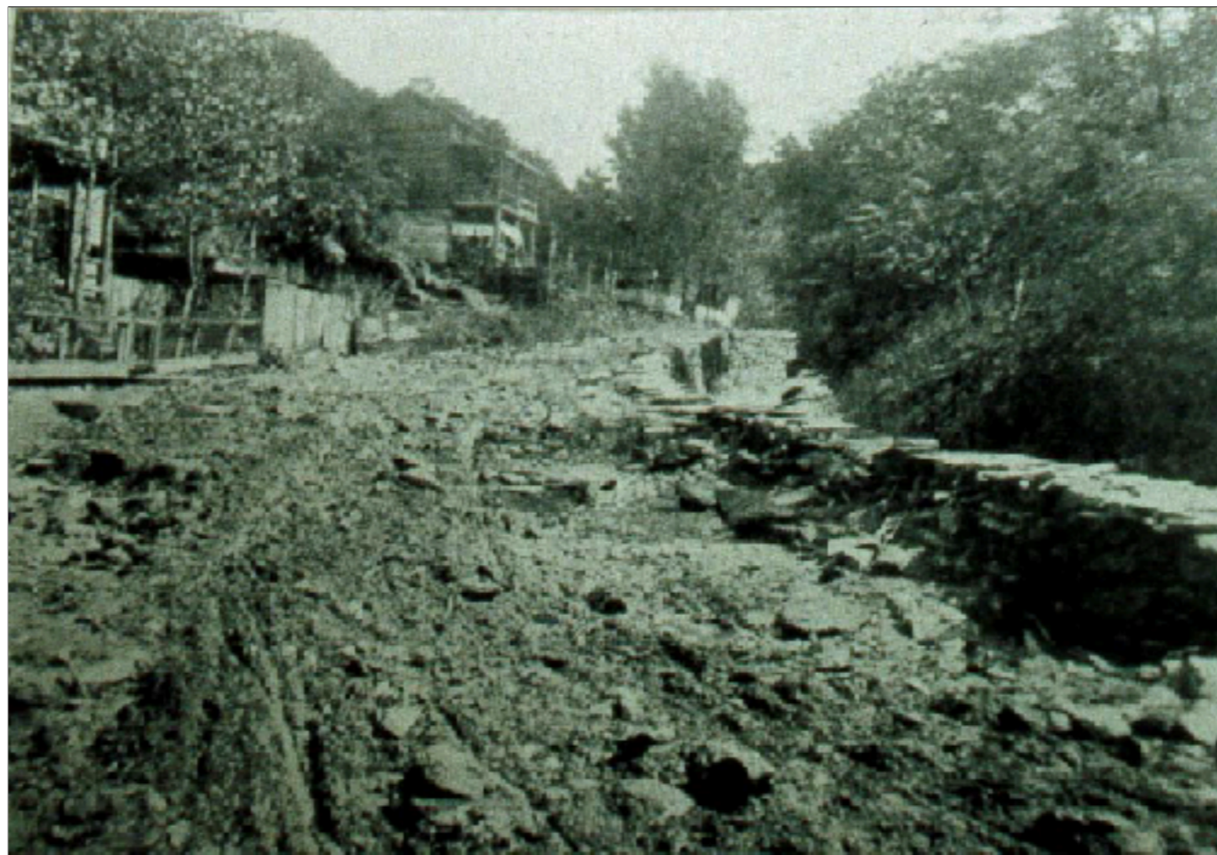
“Section of road in Amherst County before improvement.”
