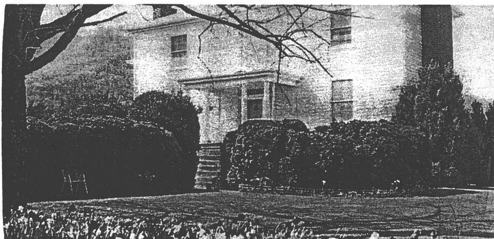
Pleasant Vale The former George Rucker place
