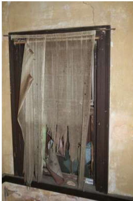
Figure 28.0- South Wall Window at Stair Landing. Room 200
