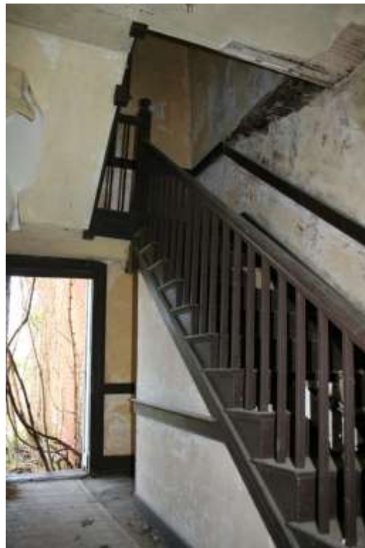
Figure 16.0- Looking Towards South Wall Door. Room 100
