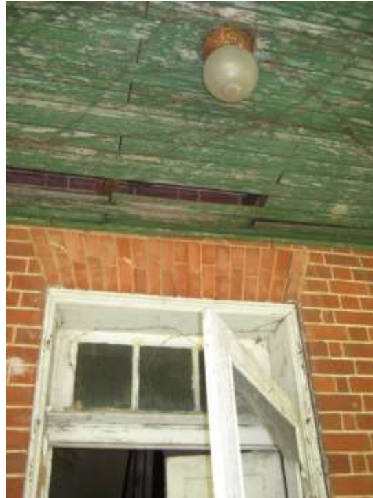
Figure 3.0-Jack Arch Above Front Door. North Facade
