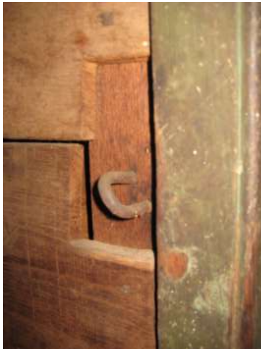
Figure 32.0- Metal Loop. Room 300
