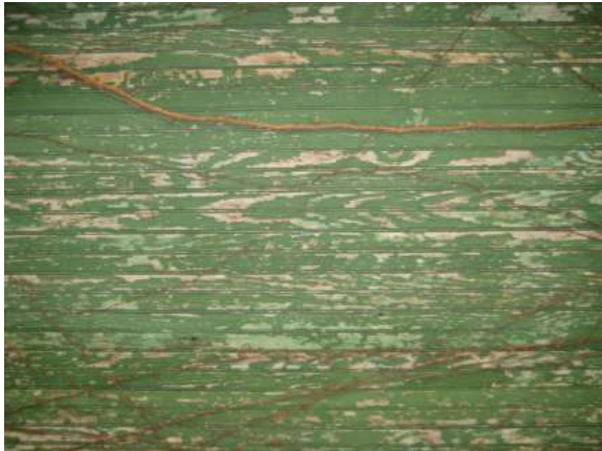
Figure 14.0- Ceiling of Porch. North Façade
