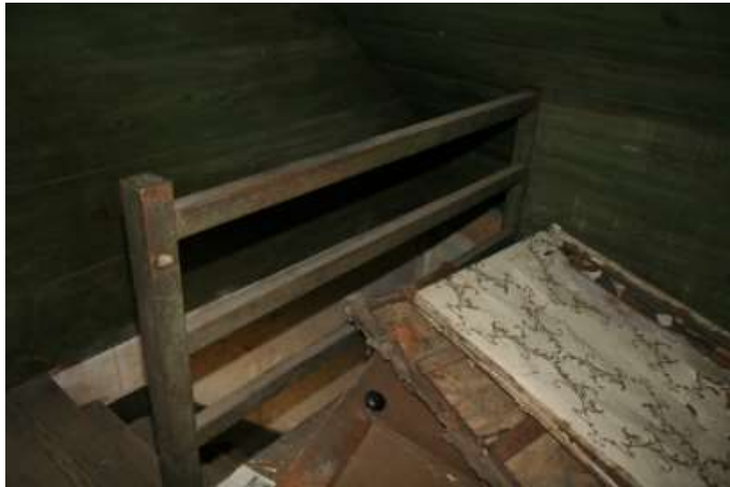
Figure 34.0- Balustrade and Newel Post. Room 300
