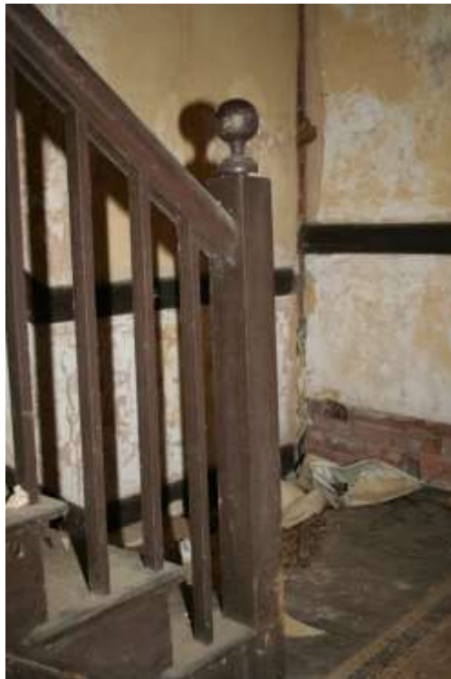
Figure 22.0- Balustrade and Newel Post. Room 100
