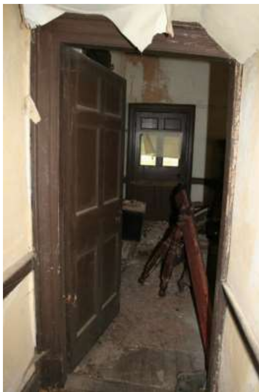
Figure 20.0- Doorway to Room 102. Room 100
