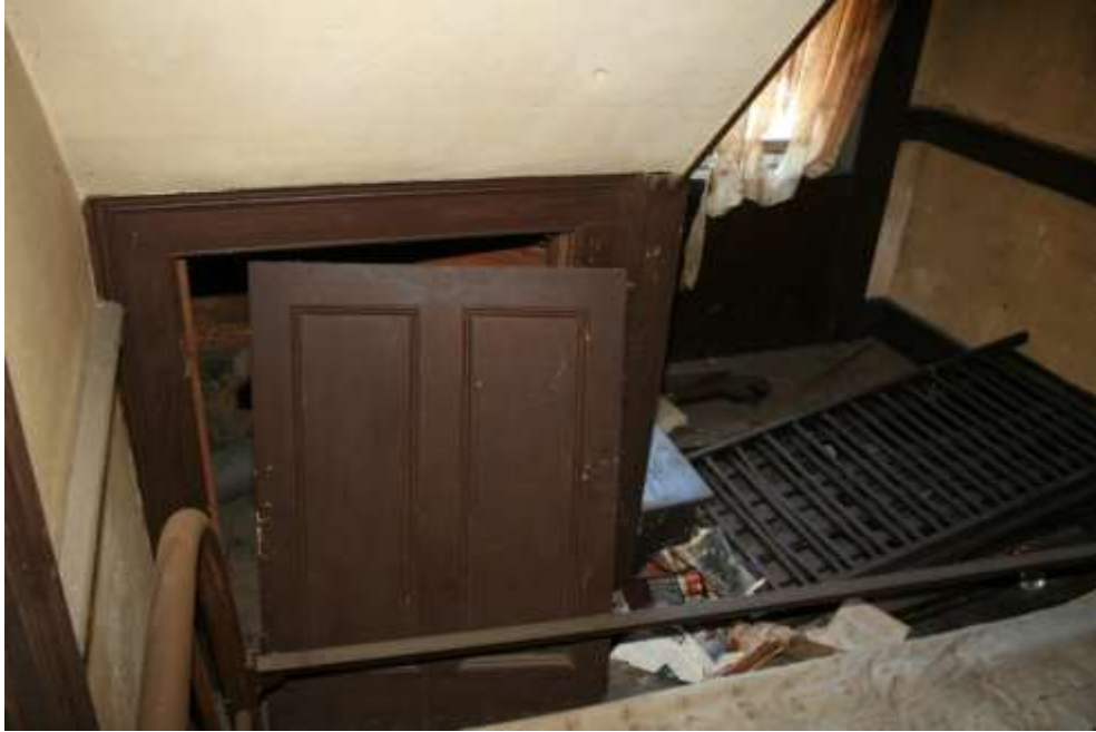
Figure 25.0- Doorway Underneath Attic Stair. Room 200
