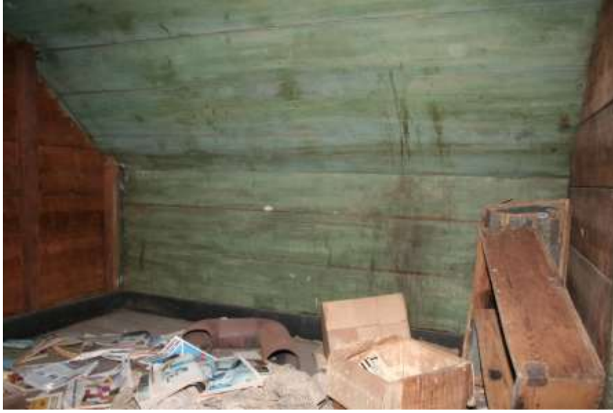
Figure 29.0- South Wall. Room 300
