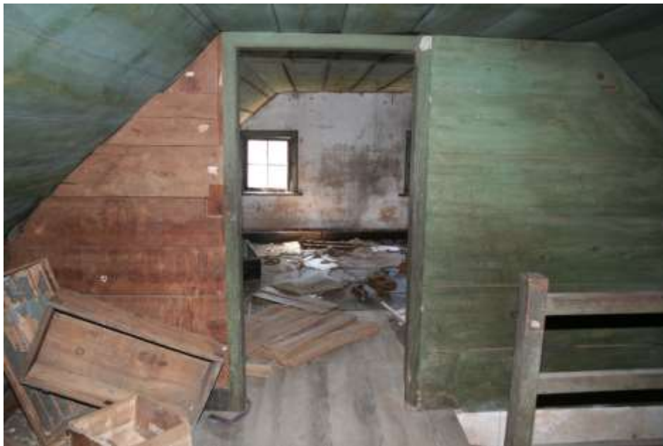
Figure 30.0- West Wall. Room 300
