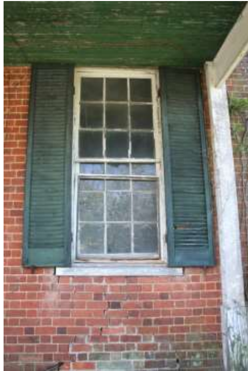
Figure 5.0-West Bay Window with Altered Mortar Below. North Façade
