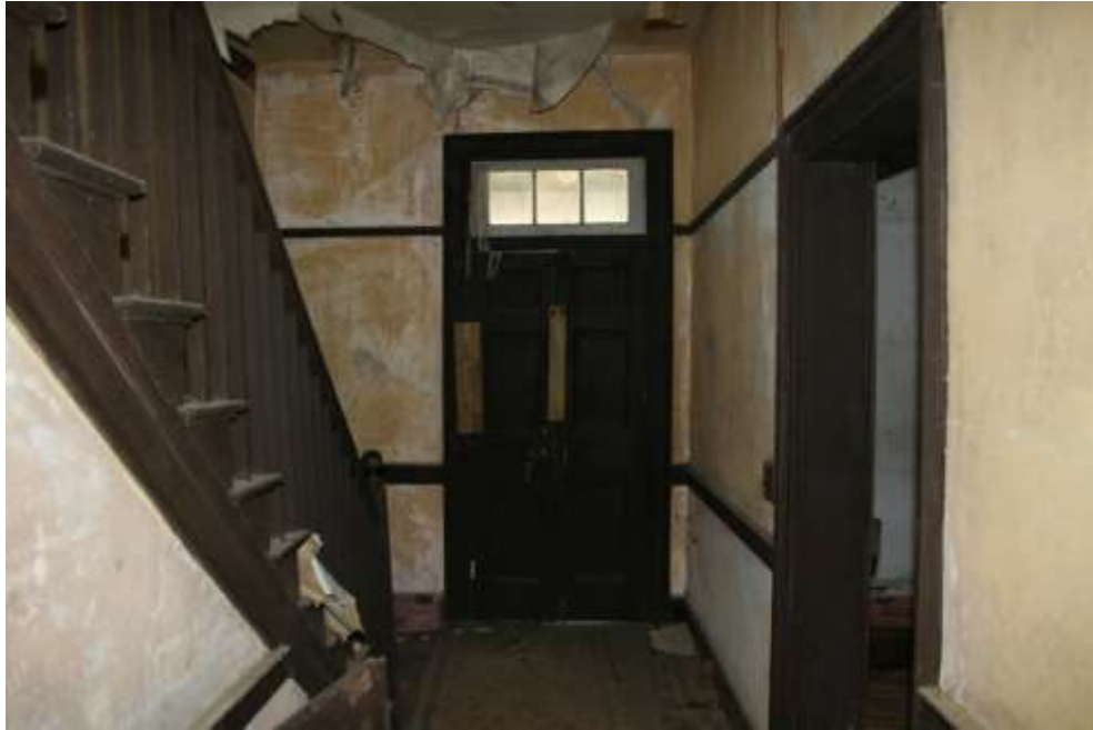
Figure 17.0- Look Towards North Wall and Front Door. Room 100
