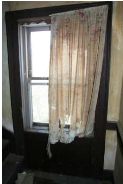
Figure 26.0- North Wall Window. Room 200
