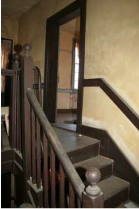
Figure 23.0- Looking Towards East Wall From Staircase Landing. Room 200
