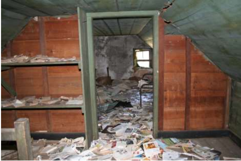
Figure 31.0- East Wall. Room 300
