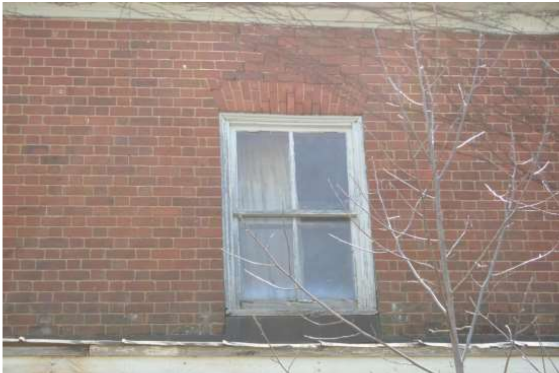
Figure 5.0-West Bay Window with Altered Mortar Below. North Façade
