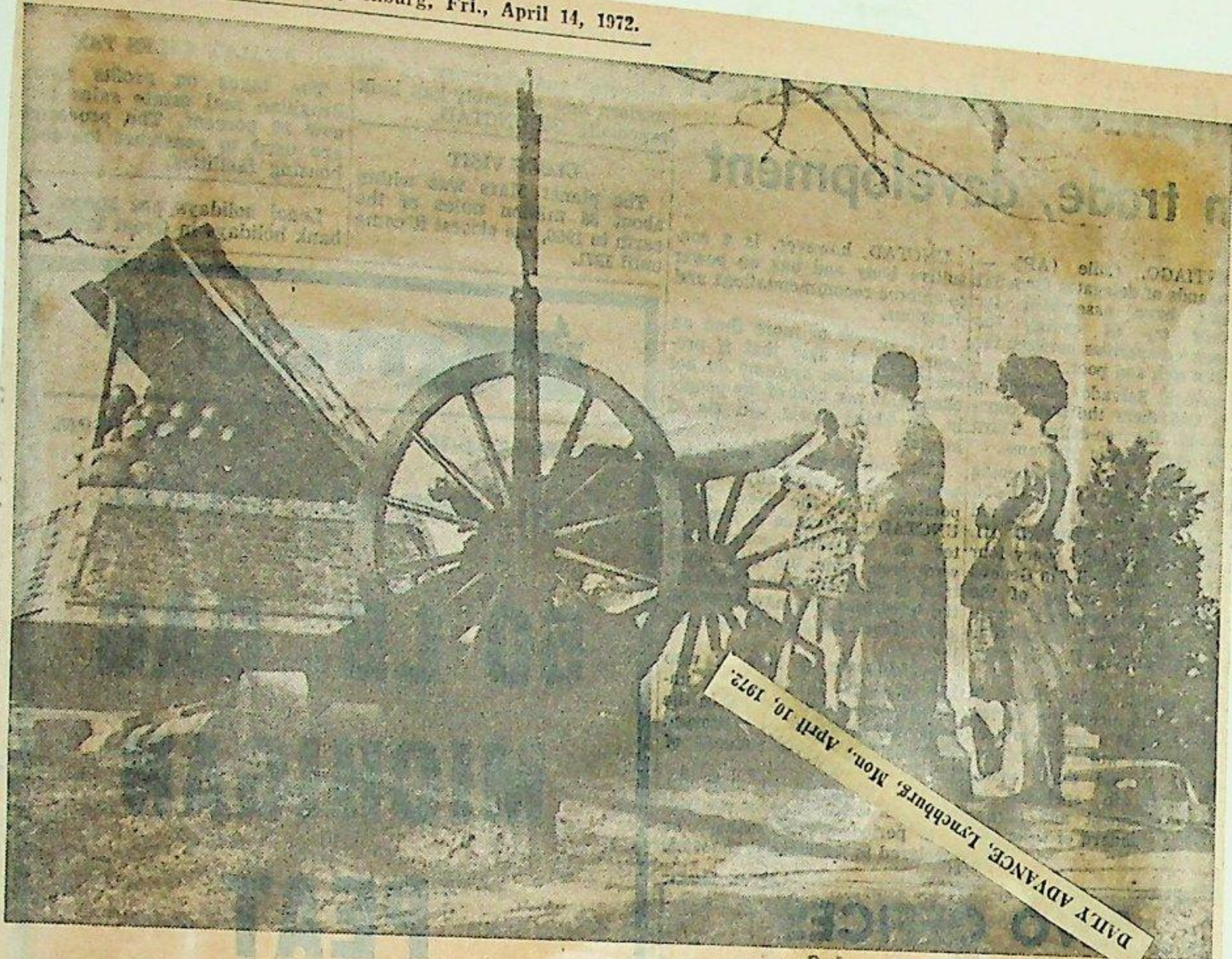
'HIGH WATER MARK'—This is the "High Water Mark" at Gettysburg, Pa., where Pickett's charge was halted on July 3, 1863. In background is the
