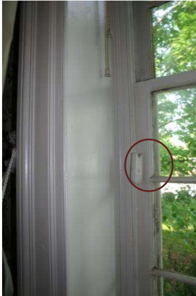
Room 102, Window 2, window sash holder (circled), T. McDonald
