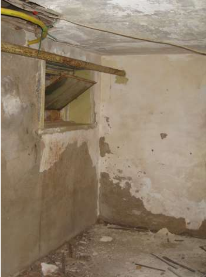
Southeast corner of room 002. K. O'Shea
