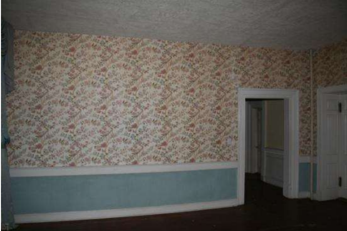
Room 102, north wall, door 1, T. McDonald
