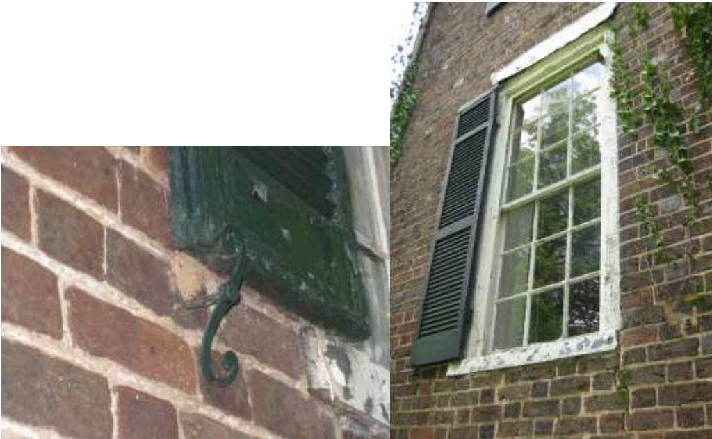
June 2008, West Elevation Shutter dog (left), and window (right), C. Lauth
