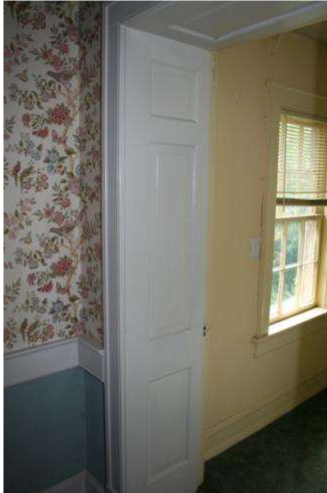
Room 102, door 3 revealing paneling in door jamb, T. McDonald
