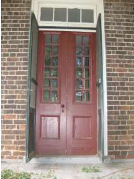
June 2008, West Elevation entrance doors, C. Lauth
