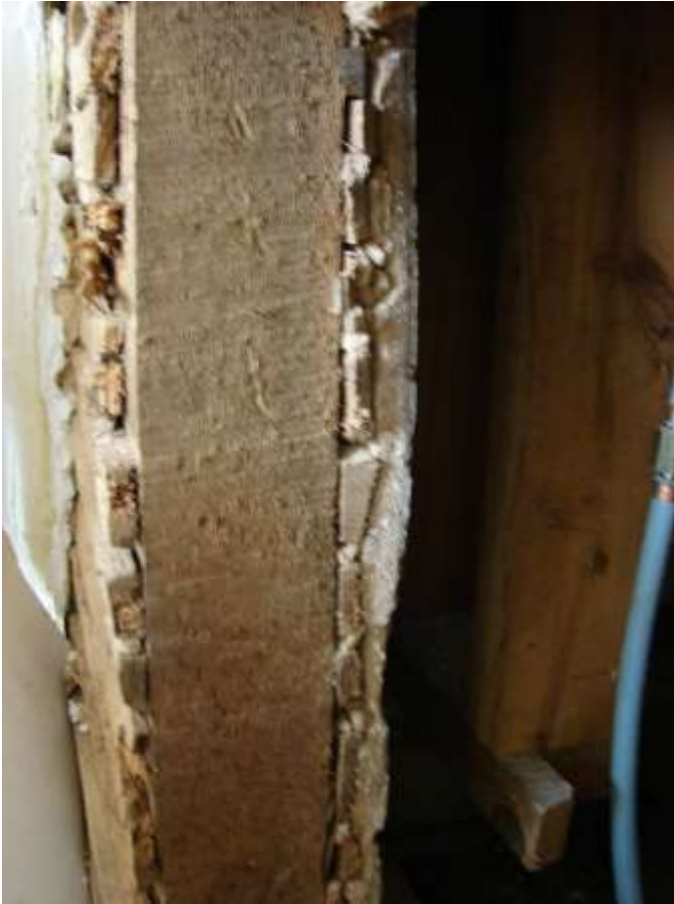
Foam insulation has been added here and a cardboard partition stapled to the original beams, which show the ghost-marks of the old laths, to cover the gap.
