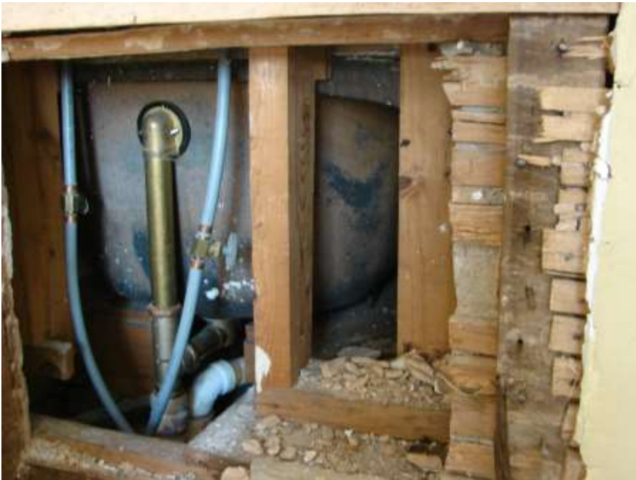
Foam insulation has been added here and a cardboard partition stapled to the original beams, which show the ghost-marks of the old laths, to cover the gap.
