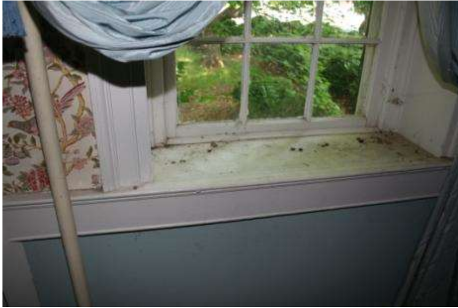
Room 102, west wall, window 1, including the surbase, the depth to the window sash is 1'2".
