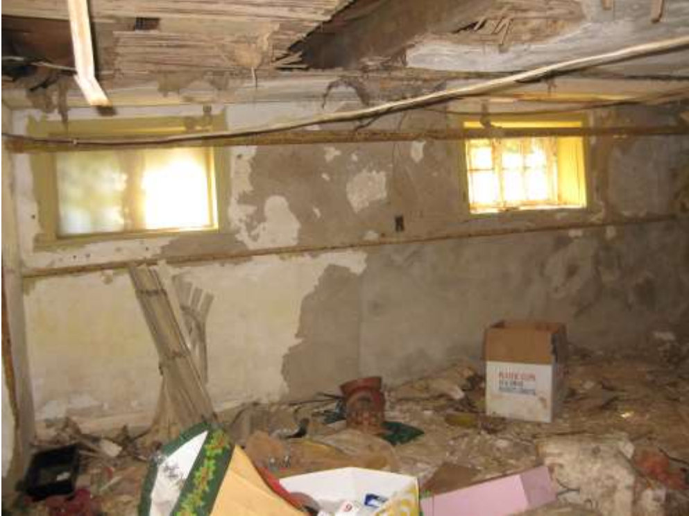
Room 002, windows on west elevation
