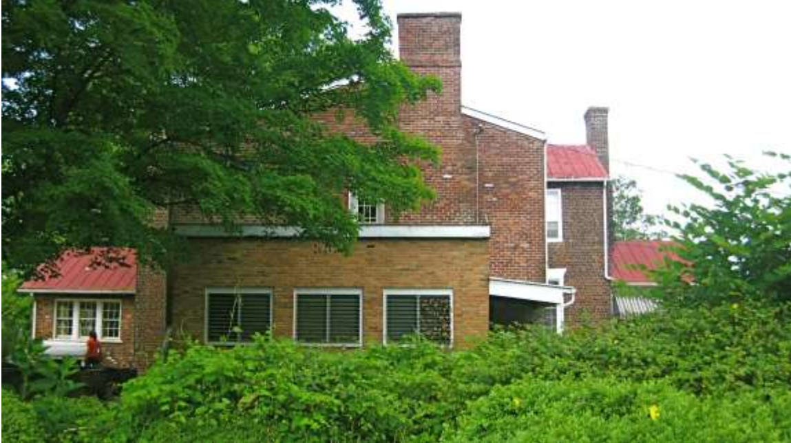
Hog Town House, May 2008, East Elevation
